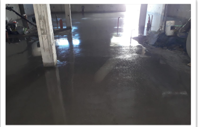
Floor is poured at Victory Baptist
