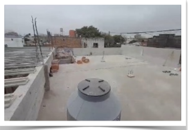
Finishing work on the roof of the church
