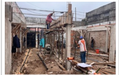
Construction of Victory Baptist
